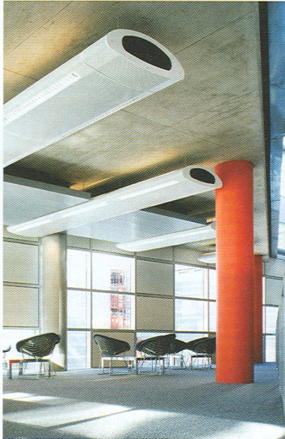
Demonstrating the capability of integrated service modules to integrate all the functions of building services and a conventional suspended ceiling into one compact unit is this installation for Imperial College in London.
