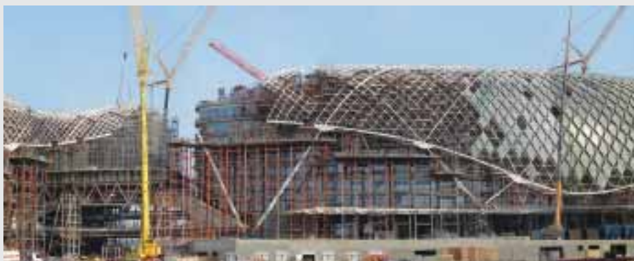
The Yas Hotel under construction in Abu Dhabi.
