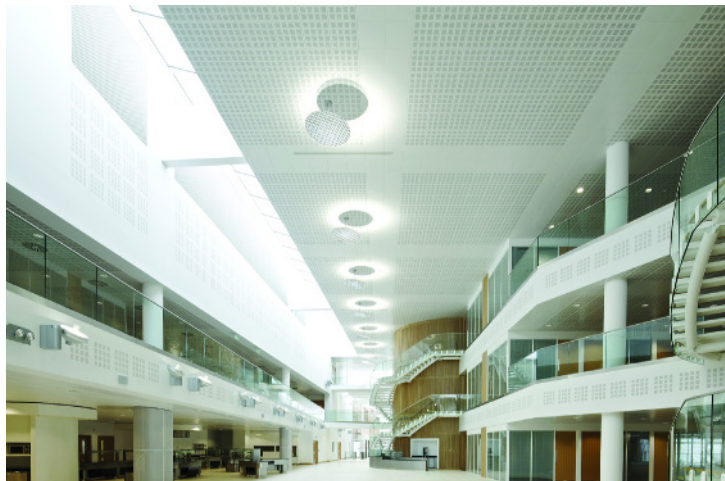
Lakeside Ceilings and Partitions' award-winning project for Ordnance Survey
