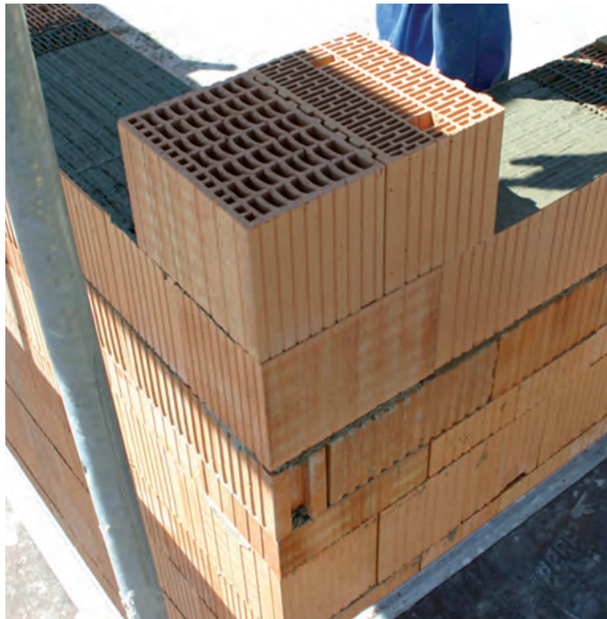
Top SAS International's C-Joint provides a tough but clear finish to partition junctions Bottom NBT ThermoPlan structural insulating blocks
