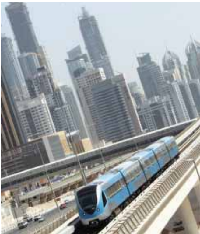
The Dubai Metro is one of VSL Middle East's key reference projects.
