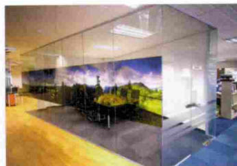
The glazing has been fitted with translucent silicone
